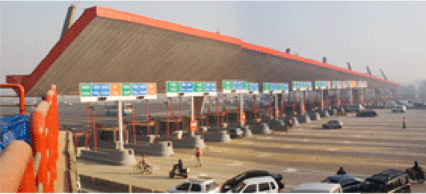
Toll Collection Systems ( TCS)
