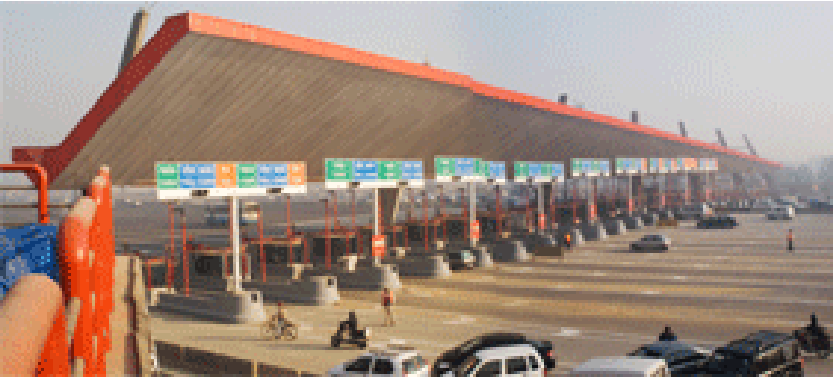
Toll Collection Systems( TCS)
