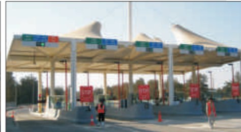
Delhi Gurgaon Toll Plaza
