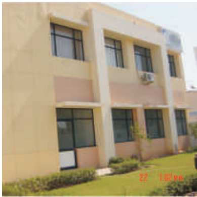
Our Works Unit at Manesar, Gurgaon.
