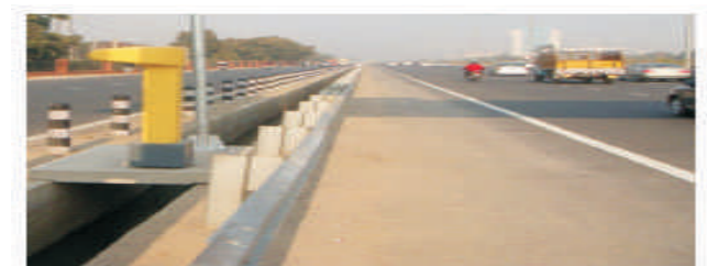
Advance Traffic Management Systems
