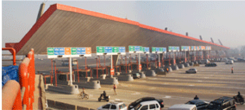
Toll Collection System ( TCS)
